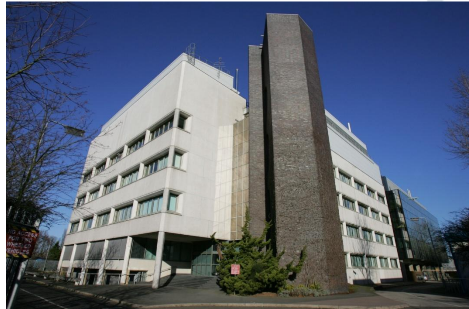
Heptares Welwyn BioPark facility
